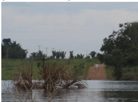
Figure 4 Flooded road in Jatuarana.
